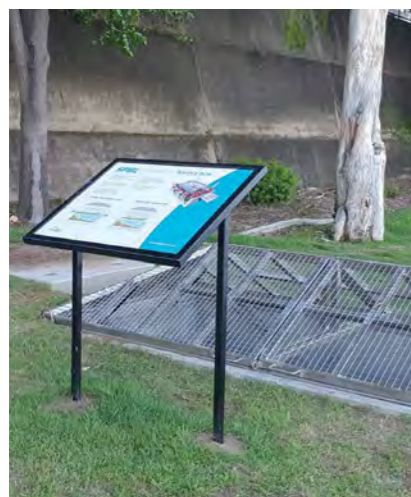
A Baffle Box installation with educational signage from another SPEL project.
