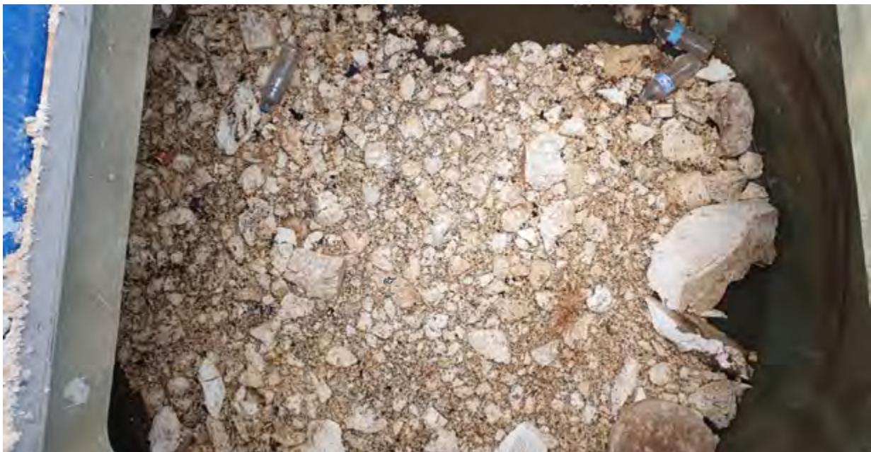
Suspended polystyrene debris inside a Vortceptor unit at Brompton Lodge
